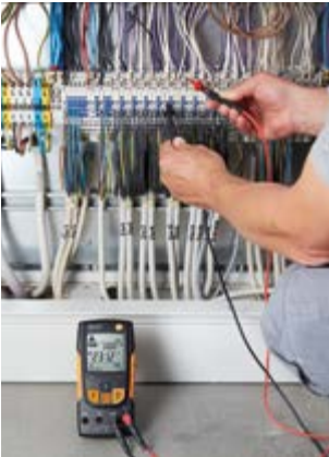
Testing voltage in a switching cabinet.
