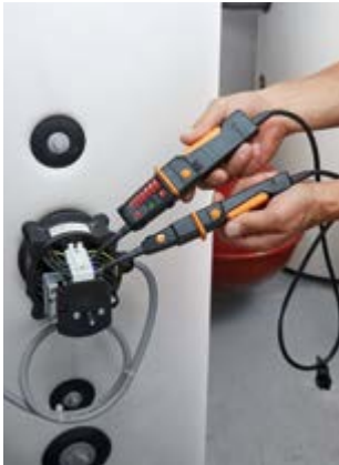
Measuring voltage on a boiler.
