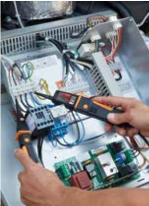
Measuring voltage on a compressor.
