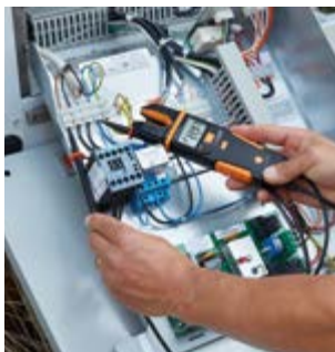
Measuring voltage on a compressor.
