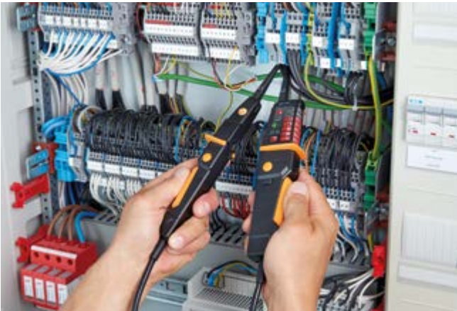
Measuring voltage in a switching cabinet.
